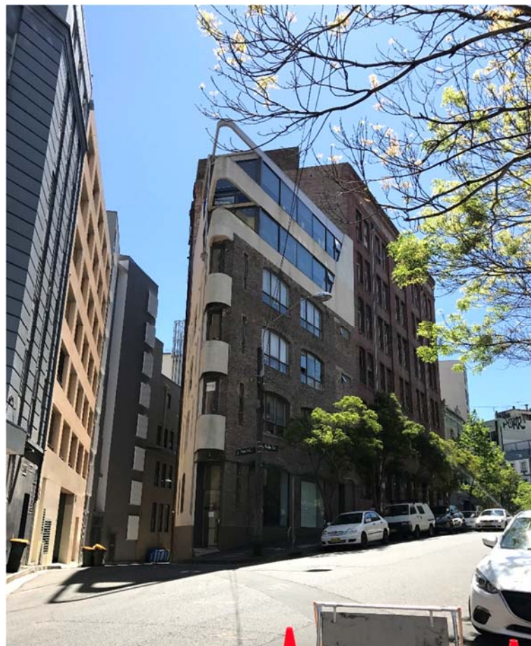
Figure 3 – Randle Street streetscape and Randle Lane corner from Chalmers Street end
