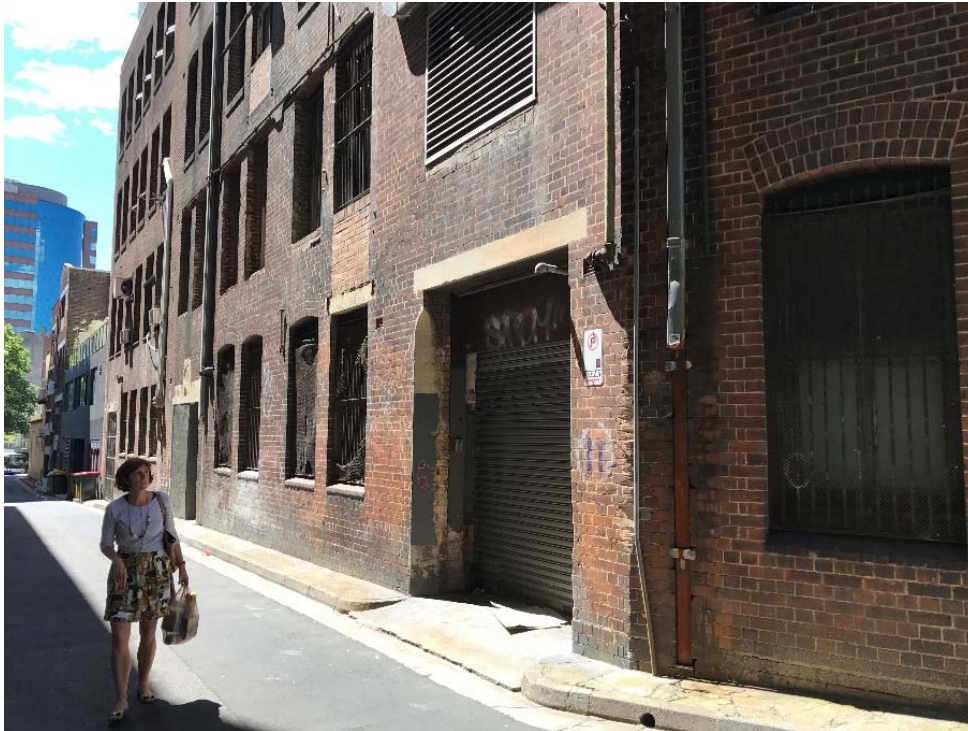
Figure 4 – Part of Randle Lane streetscape at rear of 11-13 Randle Street
