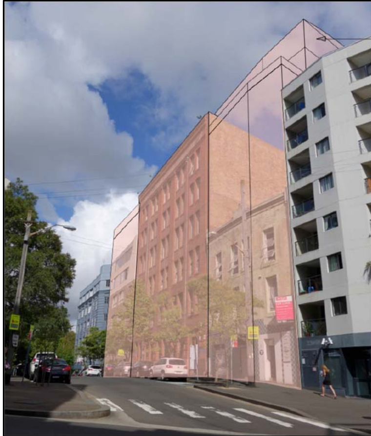
Figure 8 – Street view of proposed building envelope from intersection of Elizabeth and Randle Streets
