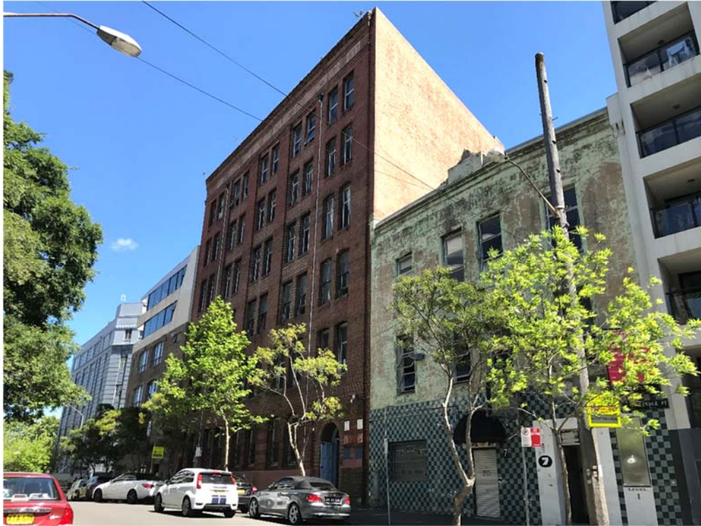
Figure 2 – Randle Street streetscape viewed from Elizabeth Street end
